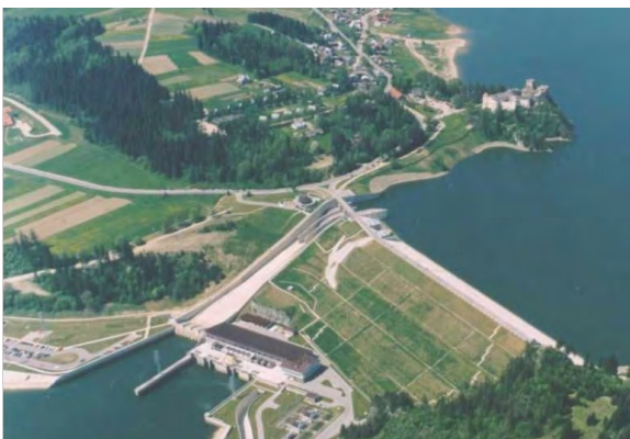
Fig. 1. The View of Czorsztyn-Niedzica dam.
