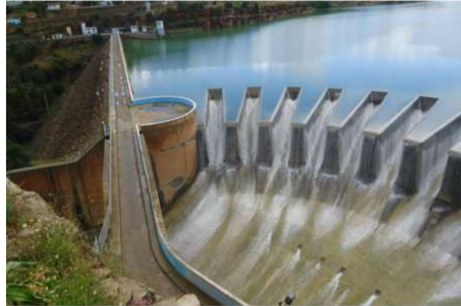
Bakhada Dam with Nonlinear weir- After 1960
