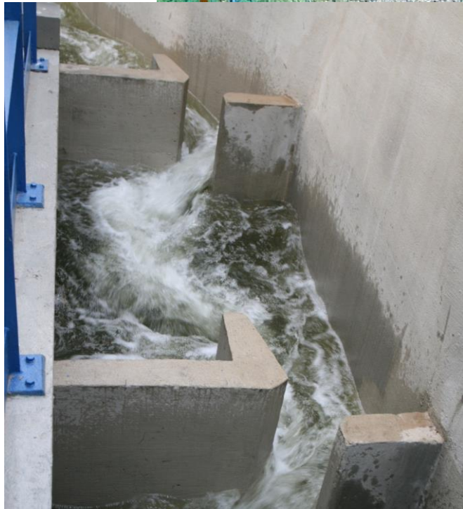
Reconstruction of the fish ladder at the Włocławek 2014. Monitoring 2014-2017.
